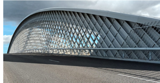
A beauty: the new "Puente de la Concordia de Valdebebas" in the northwest of Madrid.
