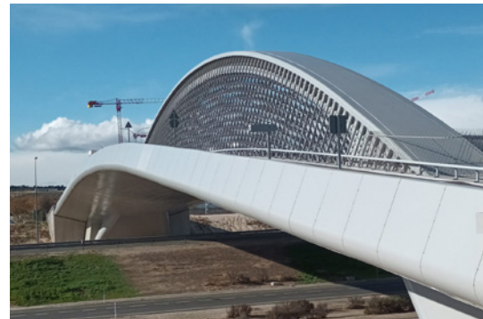
Spanning 162 metres, the arch bridge is the largest of its kind in the region.
