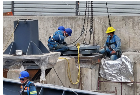
First installation of SIP®-A bearings worldwide in August 2021.
