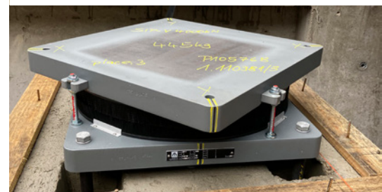
Swivelling a SIP®-V-bearing into position to protect the building core.
